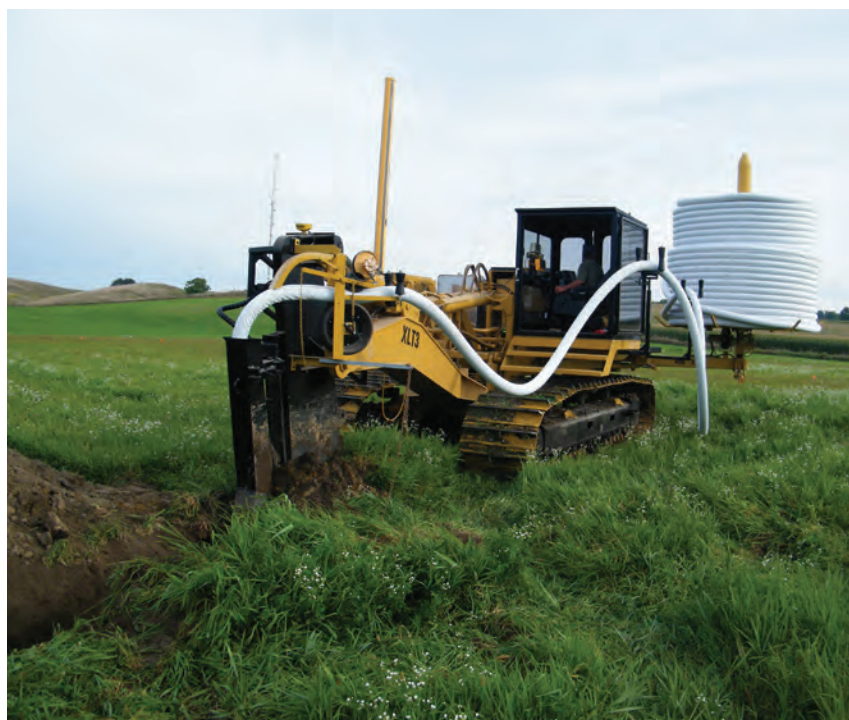
Modern drain plows can lay drainage tile with great precision.
