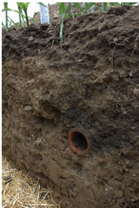
Clay tile installed below the surface of the field.
